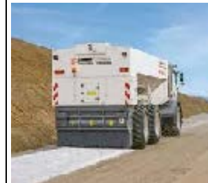
In situ application of binders
