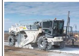
In situ mixing of binders
