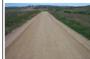
Stabilised unsealed pavement
