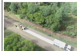
Stabilisation of unsealed pavement in progress
