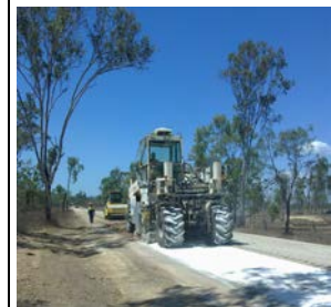
Dry spreading of binders
