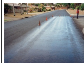
Resealing a local road
