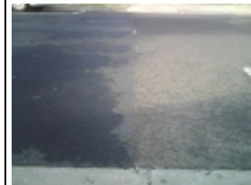
Treated and untreated surface to reduce water infiltration
