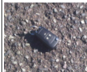
Condition at 18yrs - no treatment
