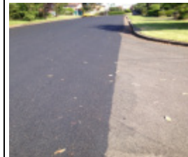
PME applied to local road to preserve ravelled asphalt surface
