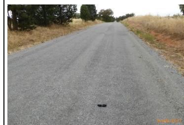
Otta seal – General view
