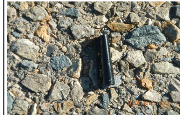
Otta seal stone grading variation
