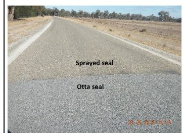
Boundaries of sprayed seal and otta seal
