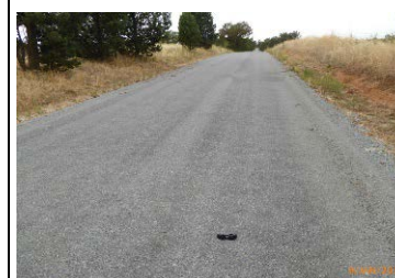
Otta seal – General view
