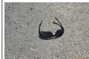
Otta seal (left) alongside chip seal
