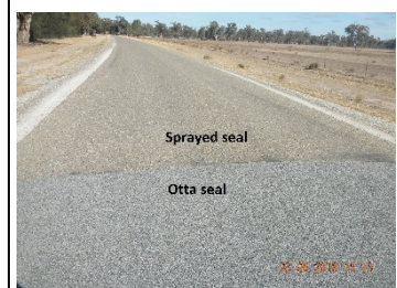
Boundaries of sprayed seal and otta seal
