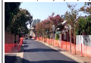
Recycled local road in Sydney
