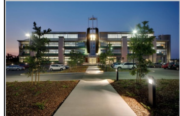
Dandiiri Contact Centre, Zillmere, Brisbane – achieved 6 Star Green Star – Office Design V2 in 2010.
