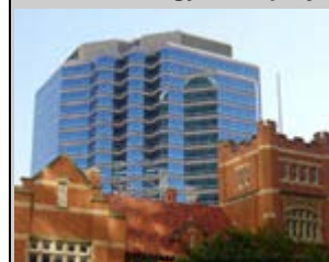
St Georges Terrace, Perth – 4 star energy rated (ABGR)
