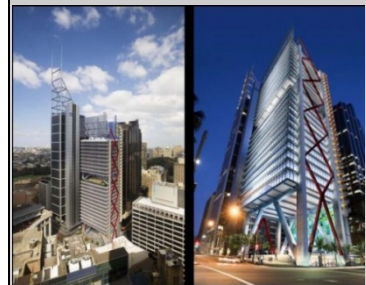
8 Chifley Square, Sydney – achieved 6 Star Green Star - Office As Built v2 in 2015.
