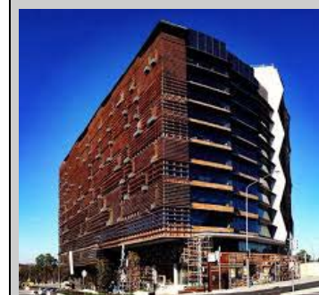
Nishi Commercial, Canberra – achieved 6 Star Green Star – Office As Built v3 in 2014.
