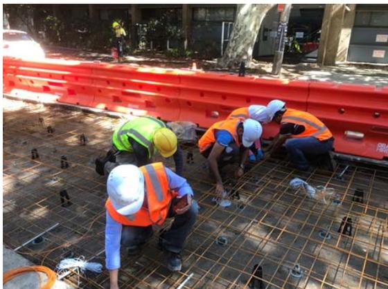
In the City of Sydney's first of its kind green road trial, they have taken industrial waste from coal-fired power stations and steel manufacturing to create a new roadway.
