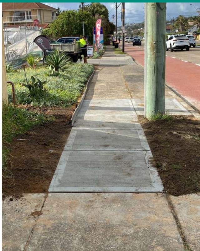
Temporary (left) and permanent restoration (right) of a concrete footpath.
