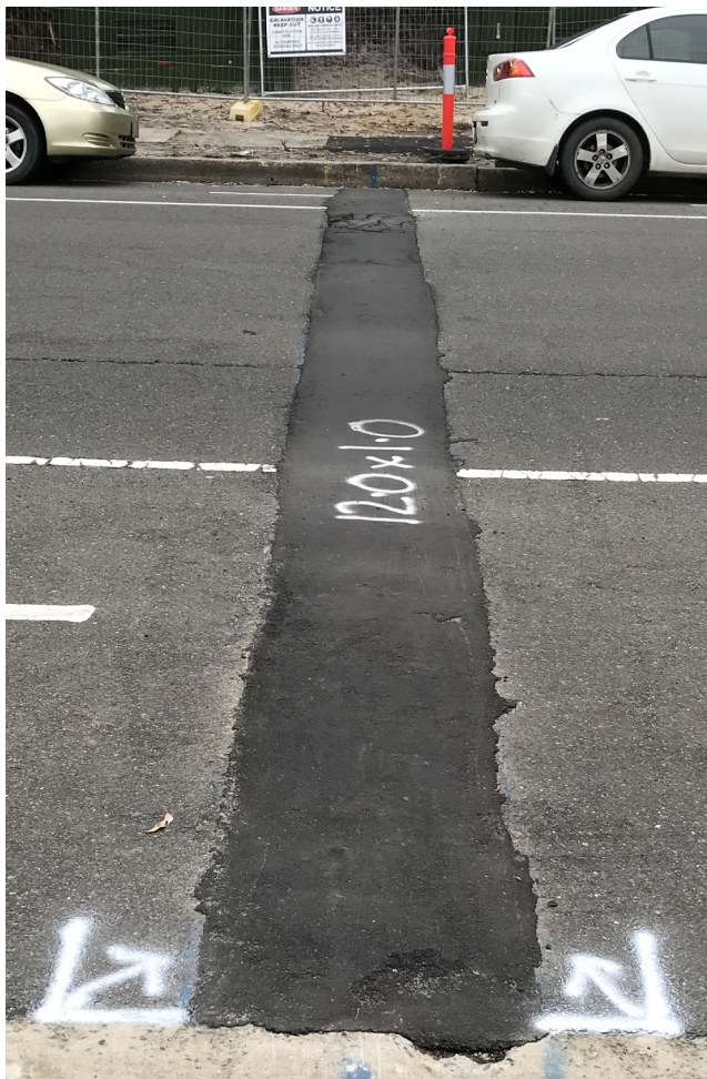
Temporary (left) and permanent (right) restoration of a trench crossing in asphalt pavement. Images courtesy of Northern Beaches Council.
