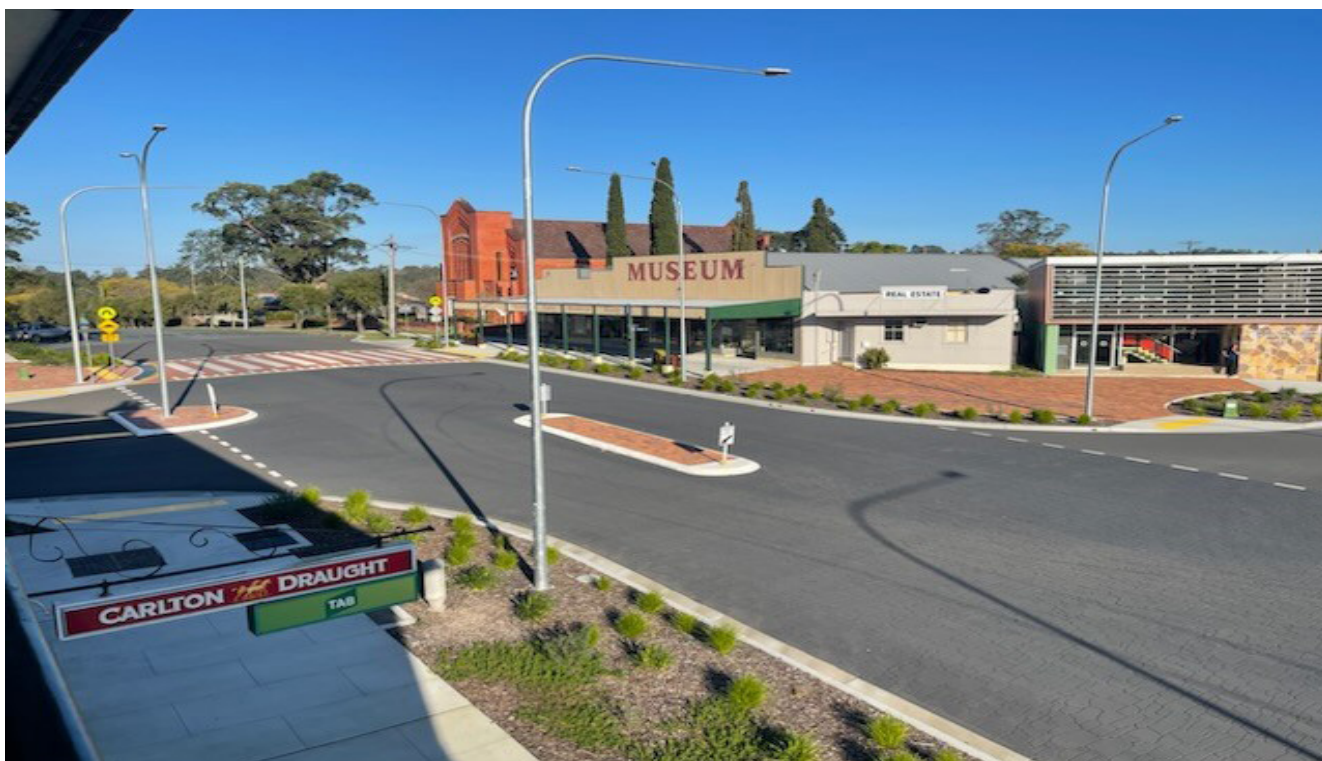
Beautification of Wingham streetscape, conversion of the Bent/Farquhar intersection to an offset T layout with enhancements to streetscape through increased sidewalk areas, specialty asphalt treatment and the undergrounding of power. Image courtesy of MidCoast Council.
